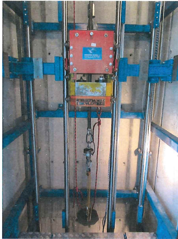
Figure 3: Configuration A (regulation system positioned at half the length of the entire device)
